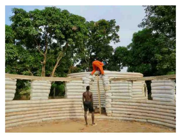
What sets earth bag construction apart is its rapid progress—an evolution unhampered by the drying time that cob demands. The ingenious technique of using bags filled with earth as building blocks removes the need for downtime, allowing your dreams to take shape with an unfaltering momentum.
